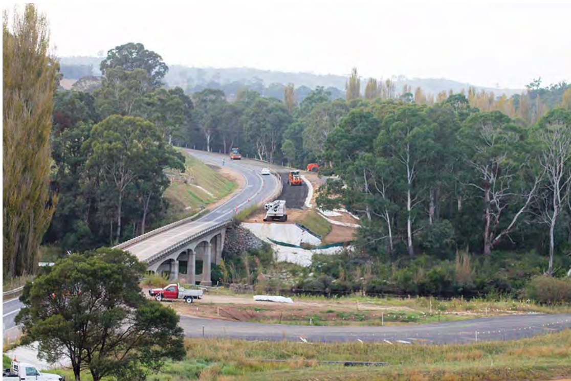
Bemboka Bridge during construction.
