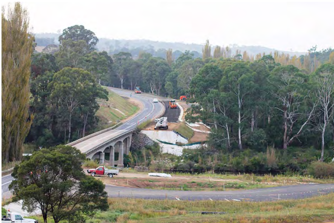
Bemboka Bridge during construction.
