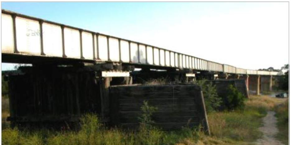
*The Gippsland Rail Needs Study notes the historic railway bridge over the Avon River at Stratford is over 100 years old and needs replacing to enable freight trains to run from Bairnsdale to Melbourne and passenger trains to travel at normal speeds. Photo taken from the Gippsland Rail Needs Study.*
