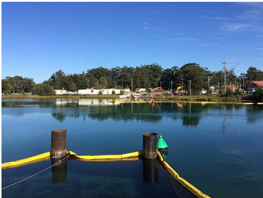
Looking south, the first pylons for the temporary bridge constructed in the channel
