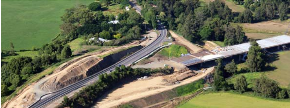
Aerial view of the works on the Foxground and Berry bypass
