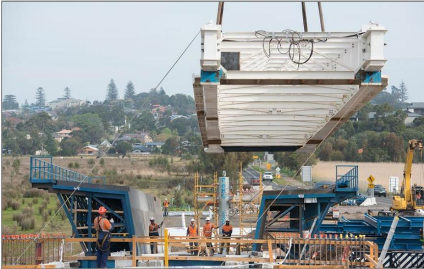
Part of the new bridge over the rail line at Fern Street is swung into place during the first stage of the Princes Hwy upgrade. The overbridge removes the rail level crossing, improving safety. Photo RMS.
